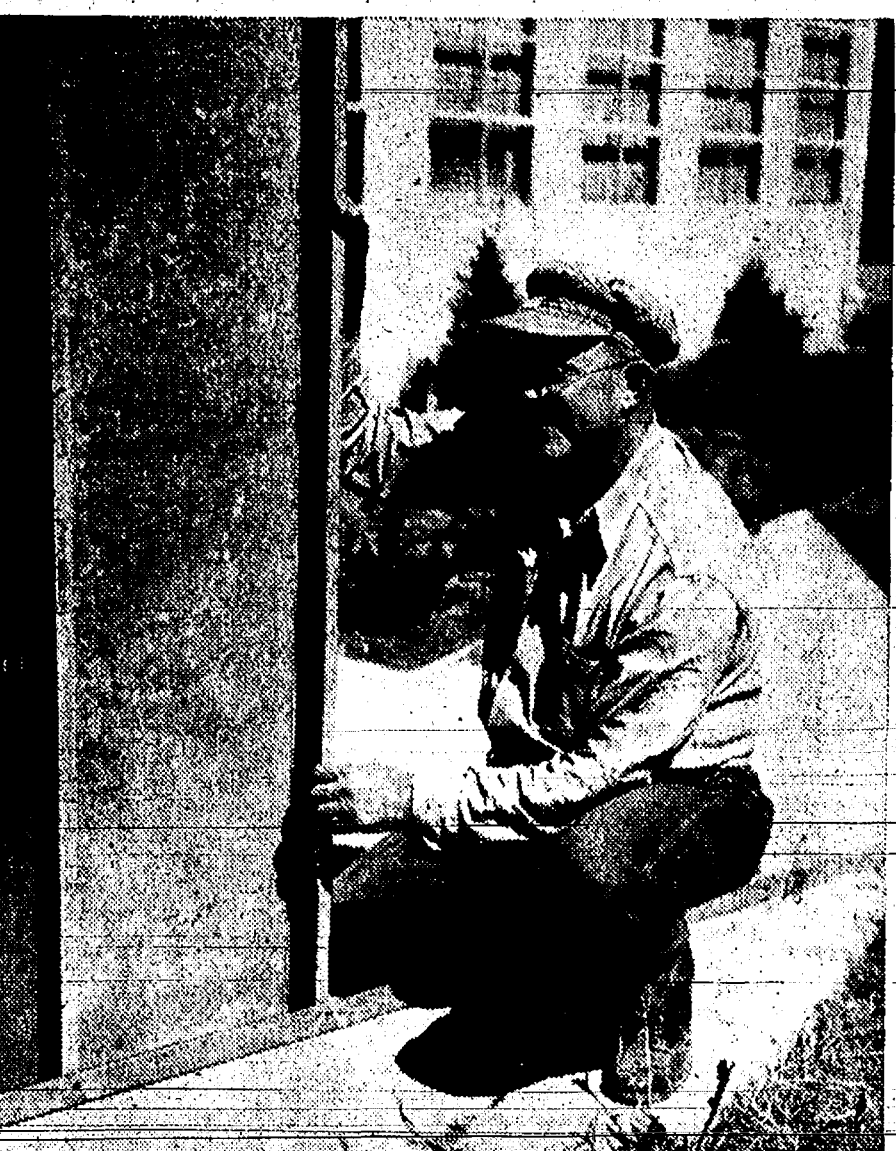
METHOD OF FASTENING steel wall panels together without nails or bolts, is shown here by Earl Beaubien, superintendent of construction on the Caro school job. At the bottom, the panels are bolted to a special angle-iron sill. In the background is a corner of the new building.
